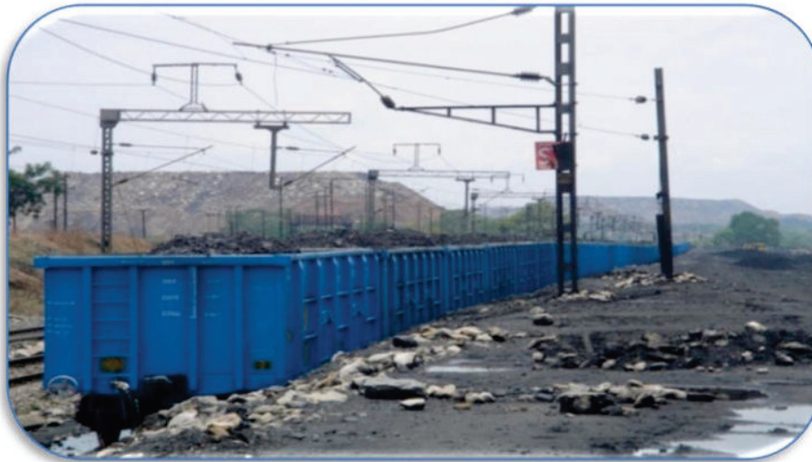
FIGURE 4.7 COAL LOADED OPEN RACK
