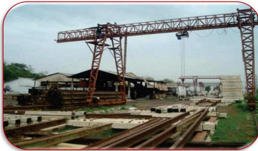
FIGURE 9.1 INDUSTRIAL MATERIAL RAILWAY SIDING
