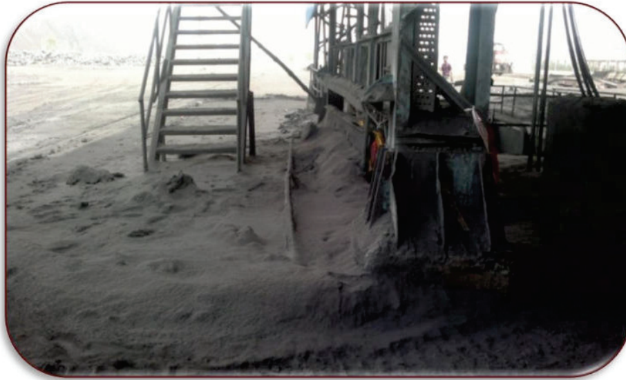
FIGURE 4.6 COAL DUST DEPOSITION AT TIPLING SYSTEM
